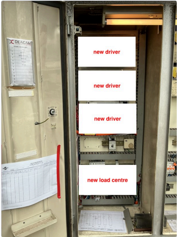
Figure 3.1 — typical existing pole switchboard section (before) and the new load-centre section fitted within the same enclosure (after).
